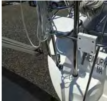
2005 C36 MKII transom design showing the compression strut positioning had fewer options due to changed stern seat design and the addition of motor mount. Note that there is also an engine hoist.
