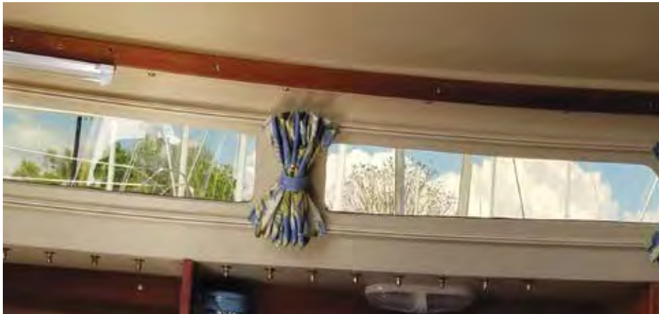
Final product from the inside, night and day from the original windows
