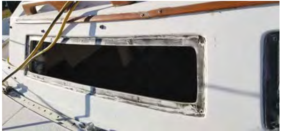
Old windows removed, some left over old caulk before final scrub
