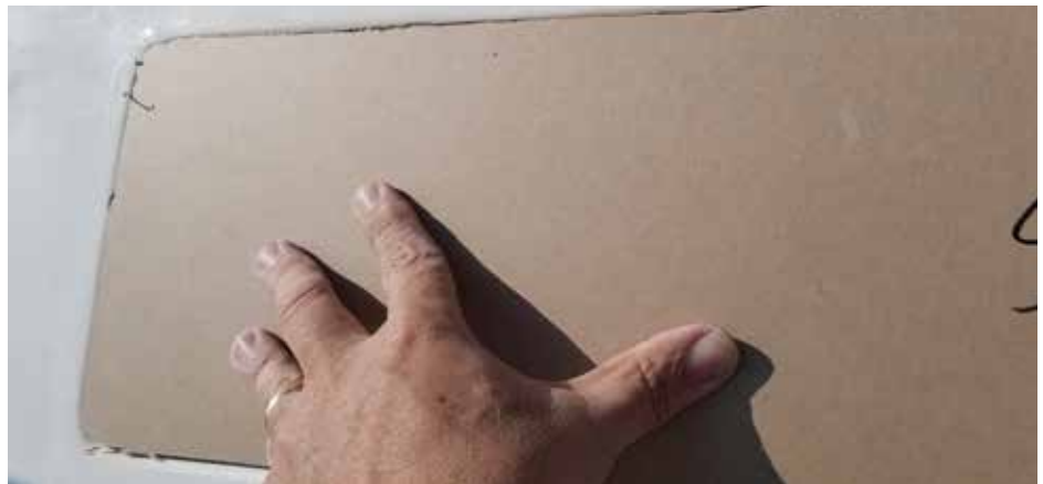
Cardboard template, cut to achieve a very tight fit
