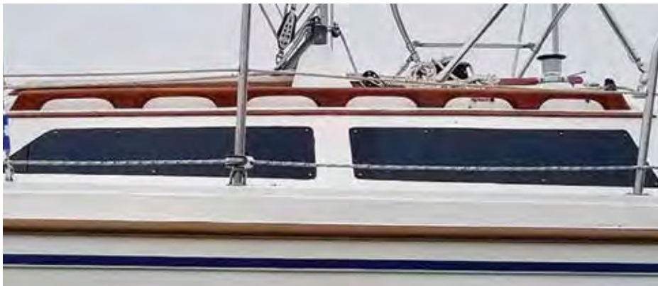
Final product from the outside, showing the new screw placements and clean lines of the caulk
