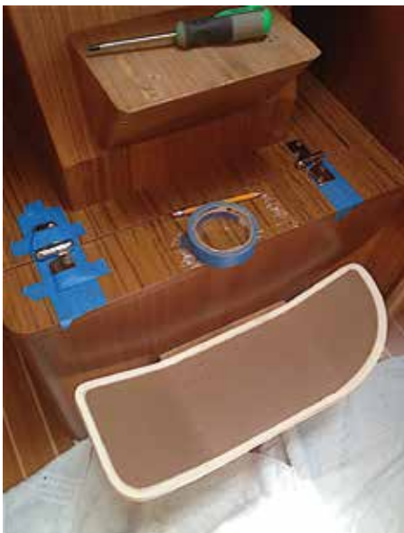
Upper and lower structures returned to normal position. Two "take-apart" hinges positioned and held in place with blue masking tape prior to being screwed in place.
